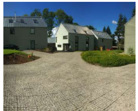
This new-build development incorporates several features to reduce flood risk. All road services are permeable (but adequate for emergency vehicles) while the rainwater that falls on the houses is taken to underground rainwater tanks to be used for WC flushing and garden use. All owners incorporated ponds into their gardens also for biodiversity reasons and car port roofs (built later) are planted to further reduce run-off.
