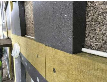
This image shows a mineral wool strip between floors to resist fire between property boundaries. Note also conduit for telecom cables is notched into the back of the insulation boards.
