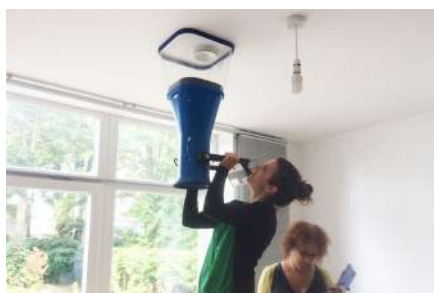
BPE: checking that high performance heat recovery ventilation systems are working as intended
