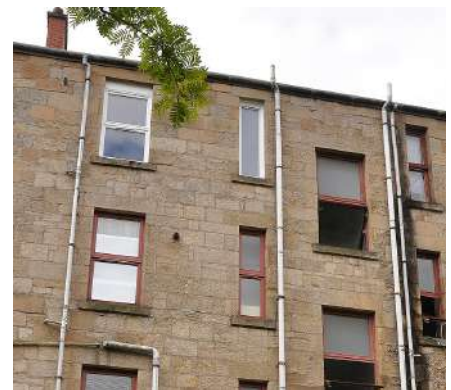
There are many issues to consider in relation to window coatings, but it is worth noting that white, opaque (paint) coatings will protect the wood better from UV degradation and thermal movement more than dark, translucent (stain) coatings
