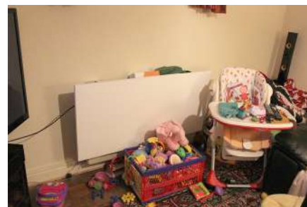
Infrared panels can be used the same as radiators but don't work as well if they are shielded from the room by furniture, as shown here
