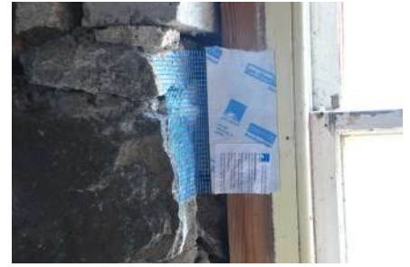
Specialist tapes like this allow for a robust and airtight seal between the window frame and adjacent plaster, but need to be installed before insulation. See [4] in both diagrams overleaf.
