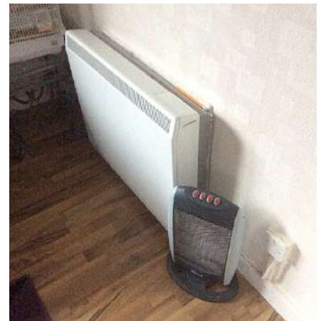
Portable heaters like this found during BPE investigations can provide evidence that the main heating system (in this case electric storage heating) is not able to maintain comfortable conditions.
